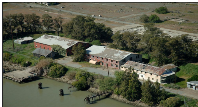
Montrose staff completed a historic properties survey as part of site assessment for the Delta Research Station on the San Joaquin River.
